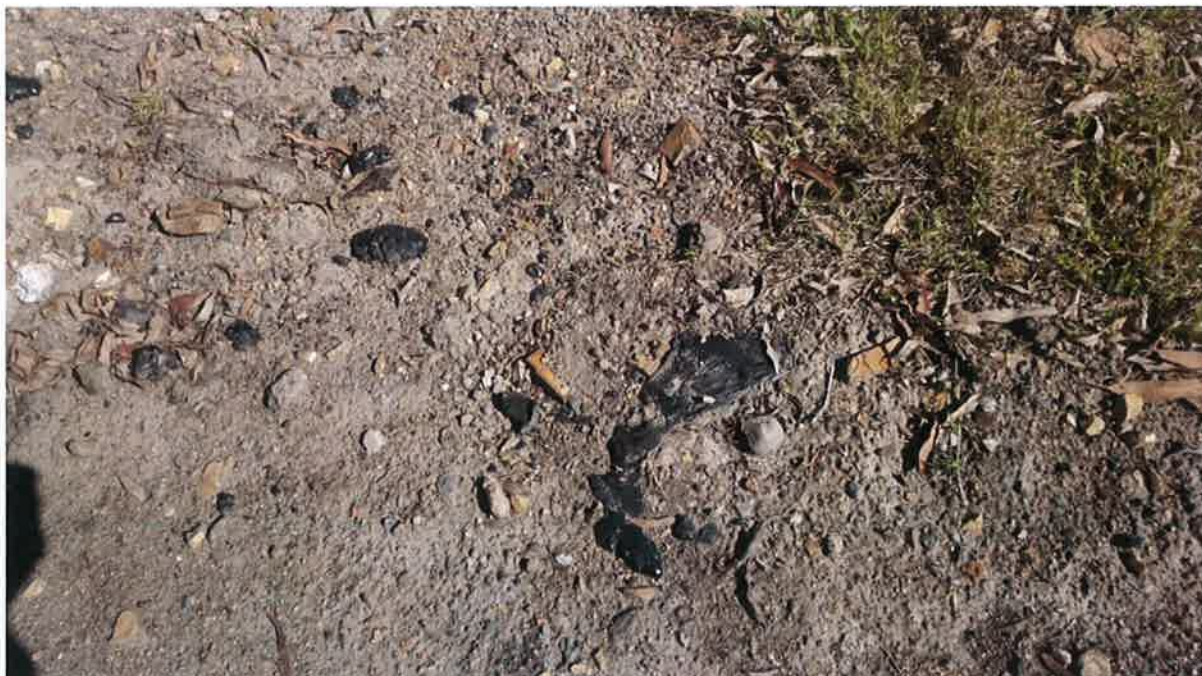
PHOTOGRAPH 4 Several tar deposits remaining on site
