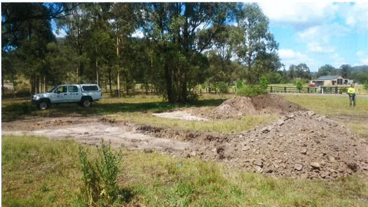
PHOTOGRAPH 3 Completed (scraped) tar impacted area showing stockpiles
