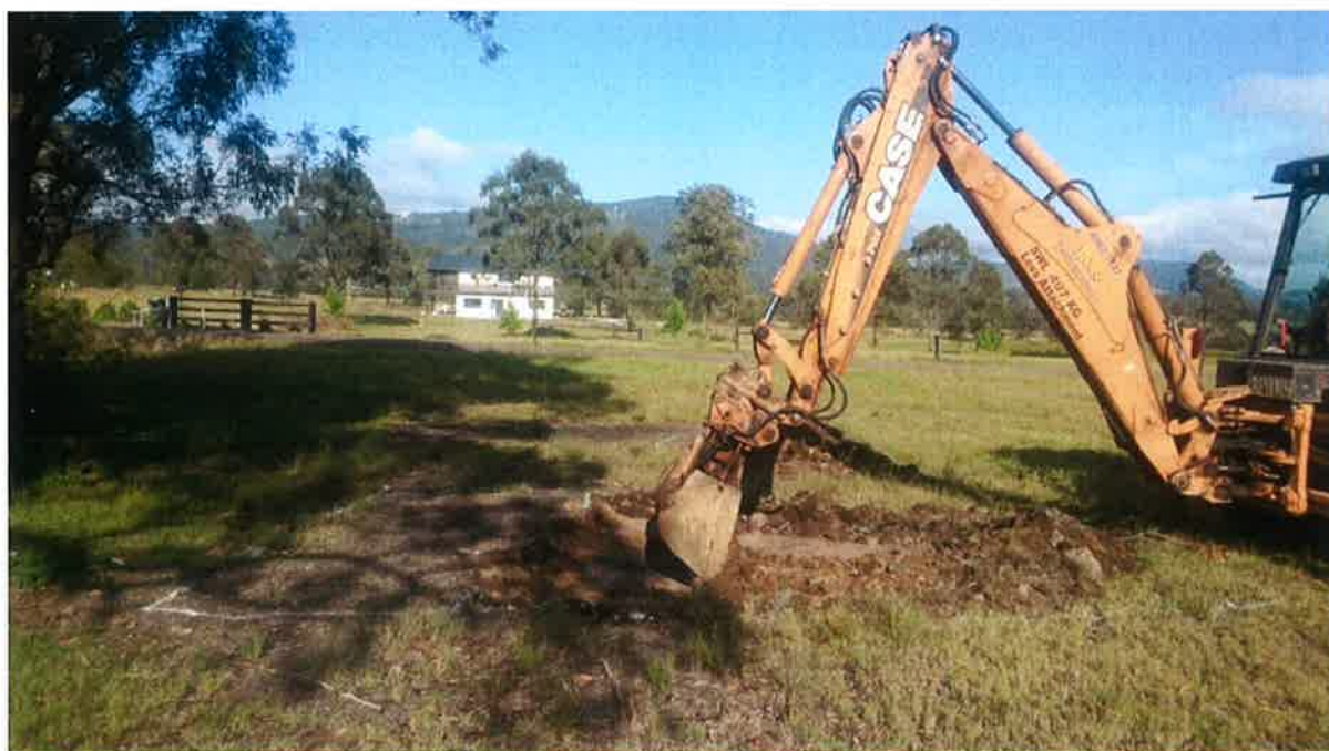
PHOTOGRAPH 2 Scraping of tar impacted area by backhoe
