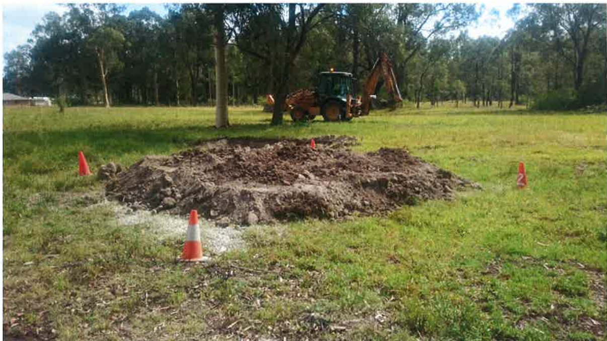
PHOTOGRAPH 6 Lime treatment area (f/ground) and location TP15 (b/ground)
